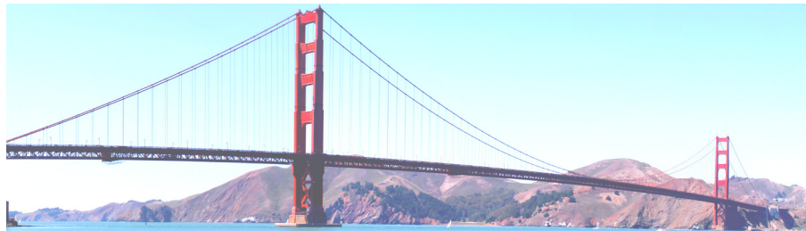
Golden Gate Bridge, San Francisco
