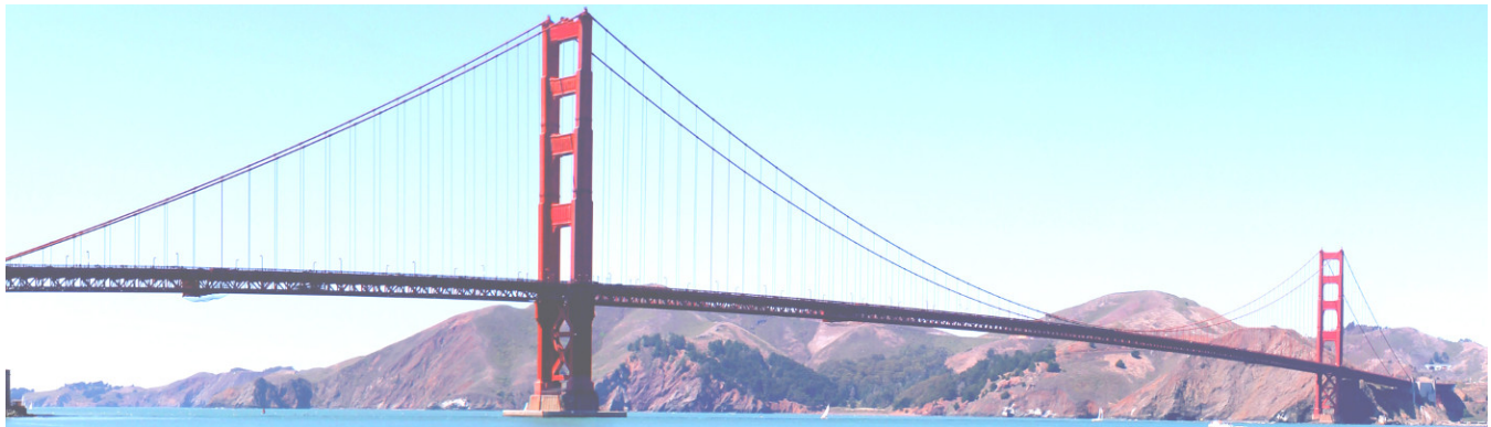
Golden Gate Bridge, San Francisco
